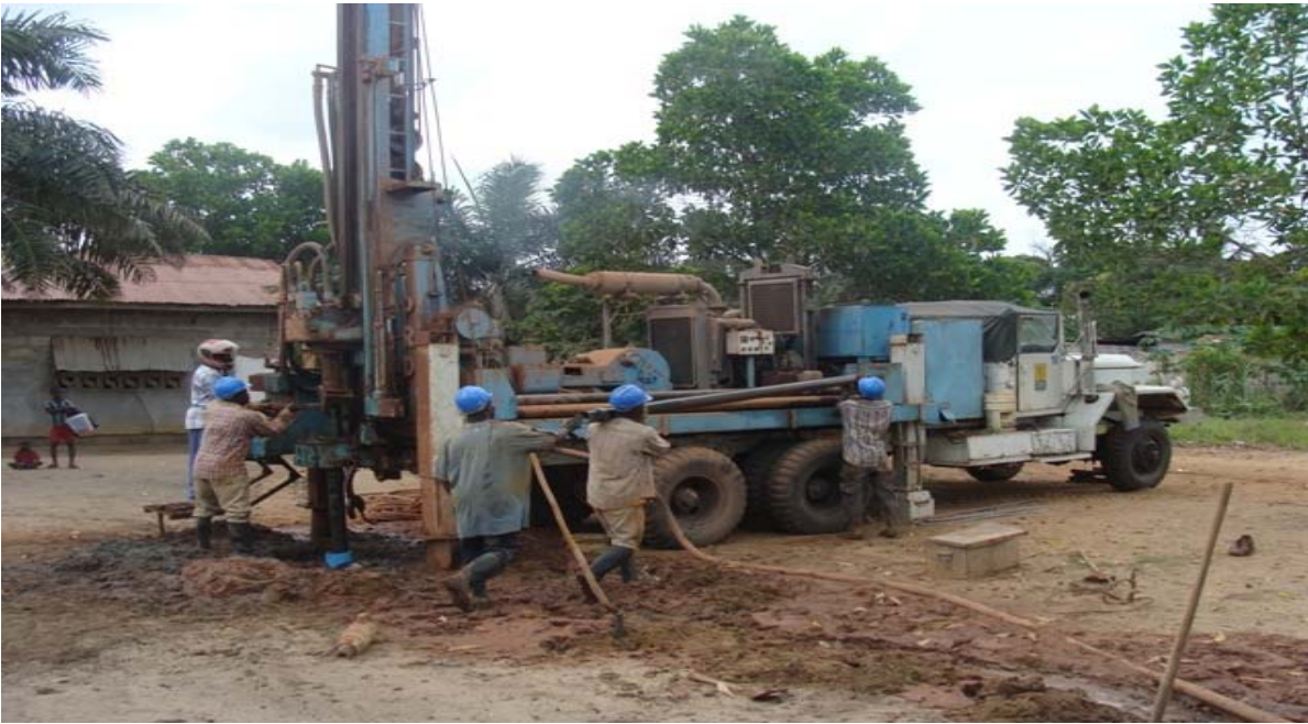
Project in Process
